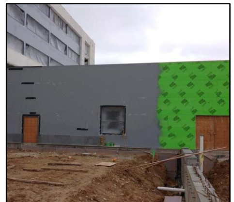
Airlok Flex ® Wall Detailing
