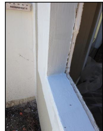
Airlok Flex ® WG window rough opening detail work using Detail Sealant PW ™
