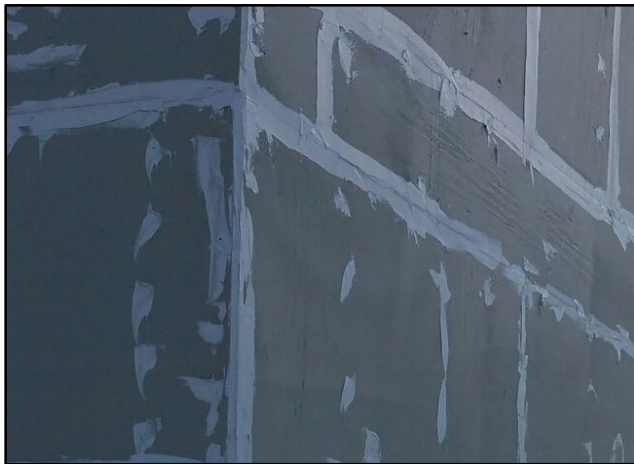
Airllok Flex ® WG field application with Detail Sealant PW ™ detail work
