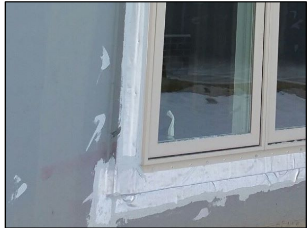
UV365 ™ Ultra Flashing (formerly Aluma Flash) at window with Detail Sealant PW ™ detail work
