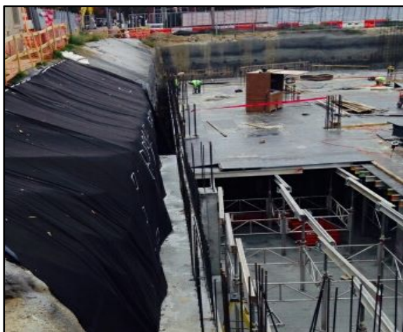
Underseal ® Blindsight ™ Membrane installation
