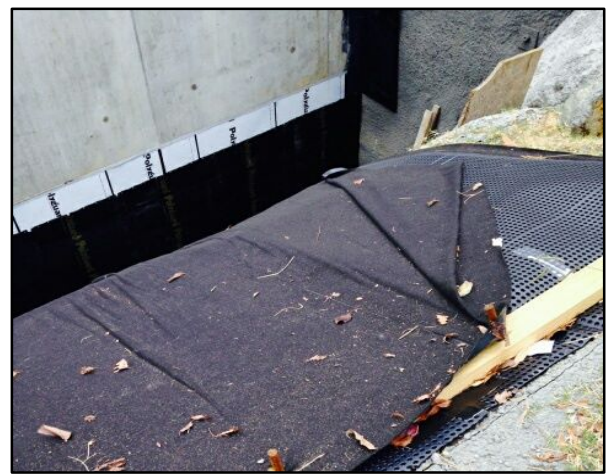
650 Membrane on concrete foundation wall covered with Polyflow ® 15 drainboard
