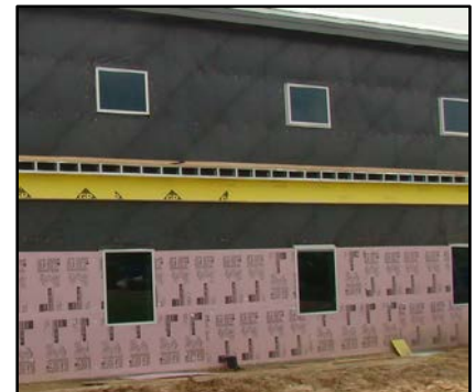
Building facade with installed windows and rigid insulation
