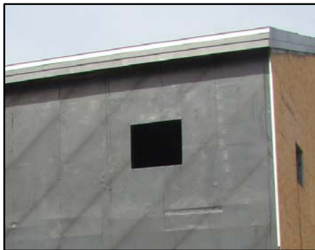
400 Membrane installation
