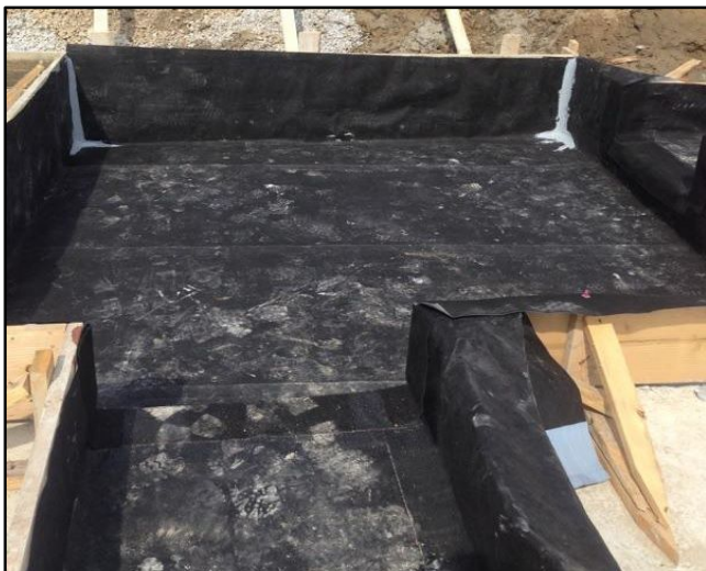
Underseal ® Underslab Membrane installation with Detail Sealant PW ™ detail work at inside corners
